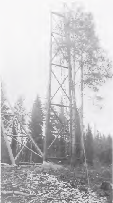
Construction of the Lenarthur Tower using winches fastened to standing trees to raise the 70 foot poles into standing position, Lac La Biche Division, Northern Alberta Forest District, 1946
