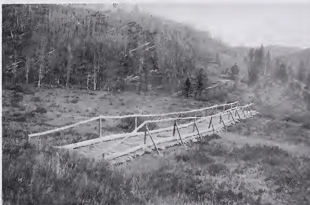
Corduoy bridge, McLean Creek, Bow River Forest, Rocky Mountains Forest Reserve, 1914. Corduoy was made of small logs laid tightly together to help horses cross soft ground
