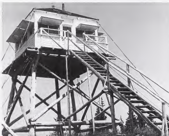
Blue Hill Lookout on wooden stilts, west of Sundre. Note wiring for lightning diffusion
