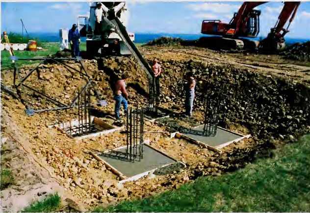
Construction of footings for the new Flattop Tower, Lesser Slave Wildfire Management Area, 2003
