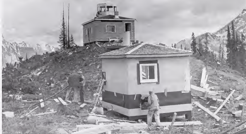
Construction of the Cline Lookout on the Upper Saskatchewan River west of Nordegg. This was the first time a helicopter was used to haul in all the materials needed. It saved many weeks of packing materials in by horse
