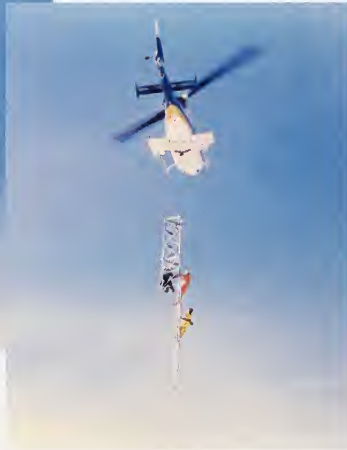
Alberta government Bell 222 C-GFSI hovering with tower section while workers bolt the sections together, 1980s
