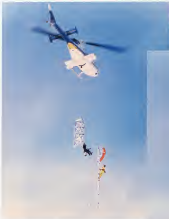
Alberta government Bell 222 C-GFSI slinging tower section to workers building single pylon tower, 1980s
