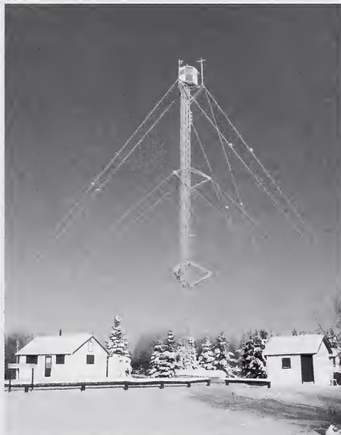
Berland Tower 110-foot single pylon construction, 1988 Alberta Government, AFHPC
