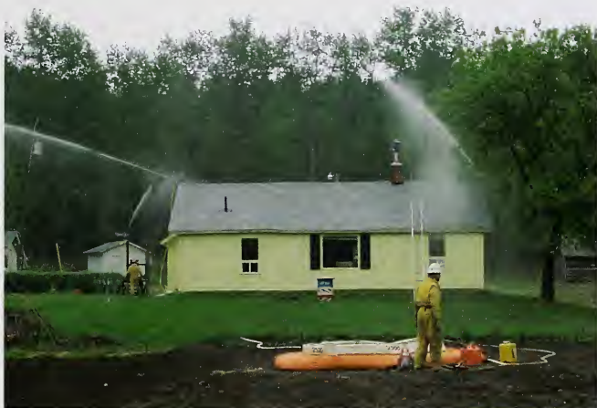
Firefighter checking pump and water supplying water to the sprinklers set up on house for structure protection, Chisholm fire, Lac La Biche Wildfire Management Area, 2001 Rick Moore
