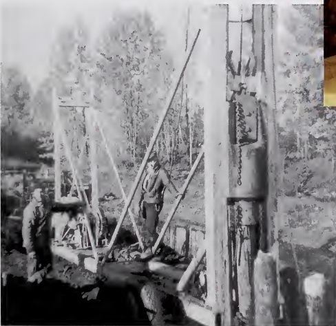
Forestry pile driver being used for the construction of the first bridge over Tony Creek (west of Fox Creek) on the Tony Tower forestry road. Pile driver was built by AFS mechanic Ray Kimzey. Raymo Quaranta and Allan Wagner operating the pile driver, Whitecourt Forest, 1959
