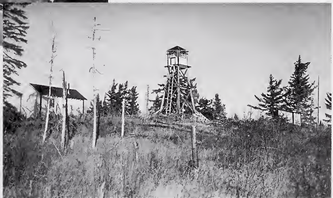
Whitecourt Lookout, 1938. This 10-metre tower was built with local timber
