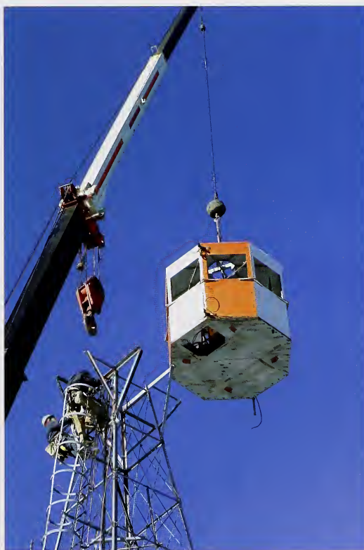
Cupola exchange on Pass Creek Tower, 2004, Whitecourt Forest
