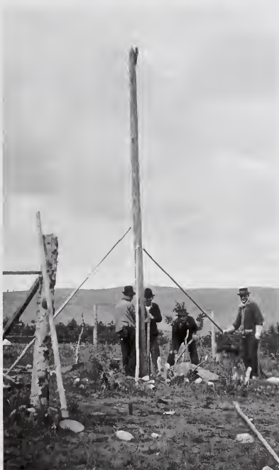
Rangers install first pole on the North Trunk Telephone Line. Phone lines were a vital link for rangers between their cabins, headquarters and lookouts. Bow River Forest, Rocky Mountains Forest Reserve, 1922 Dominion Forestry Branch, AFHPC
