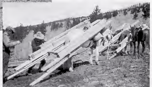
Grueling duty - horses drag lumber to summit for construction of Coliseum Lookout, near Nordegg, Clearwater Forest, 1927. Hauling lumber by this travois method was easier on the horses than the tandem method, but needed a wider trail
