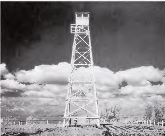
McLennan Crawl Tower, 1965. This native timber structure enabled the ranger to ‘crawl’ up for a look around his area
