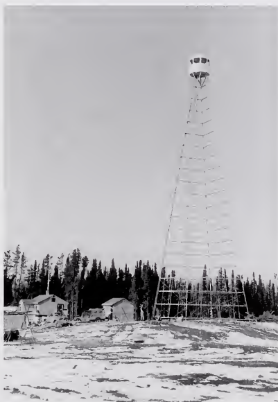
Typical construction and layout of tower and cabin Alberta Government, AFHPC
