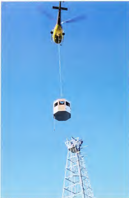
Cupola exchange completed by A-Star helicopter at Pinto Tower, Grande Prairie Forest, 1997
