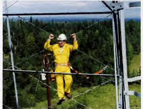
Darryl Johnson, Forest Protection Technician, climbing down outside Pass Creek Tower checking tightness of bolts on tower legs and cross pieces. Generally a crew of four to five Forest Officers would work on the tower. Fox Creek District, Whitecourt Forest, 1991
