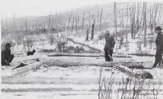
Crew lays first round of logs for the Moberly cabin, a ranger station on the Lower Trail north of Entrance. Note fire-damaged forest in background, 1939
