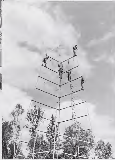
Construction of steel tower. Prefabricated cupola to be placed on top Alberta Government, AFHPC
