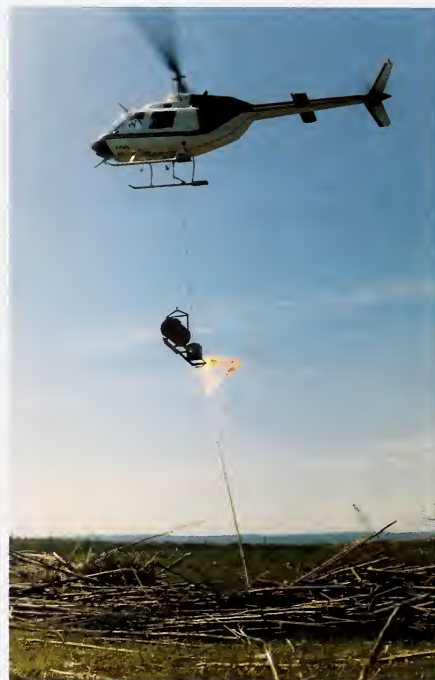
Alberta government Bell 206B registration C-FAFL lighting piles with aerial torch, 1980s
