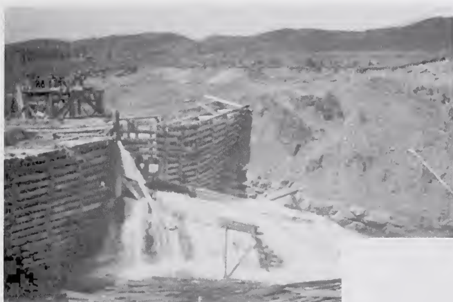
Eau Claire and Bow River Lumber Company log drive - sluicing logs through the lower dam on North Ghost River, 1924
