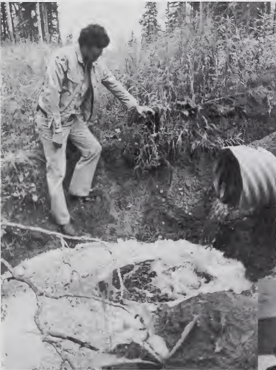
Ranger Gary Mandrusiak checks poorly-installed culvert. 'Hanging culverts' are barriers to passage of fish and other aquatic life Alberta Government, AFHPC
