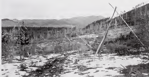
Poles used to build tripods in the construction of telephone line system. Construction of phone lines through open areas like this lessened maintenance caused by trees falling across the line. Bow River Forest, Rocky Mountains Forest Reserve, 1920s Dominion Forestry Branch, AFHPC
