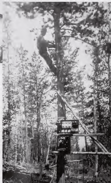
Temporary field telephone installation, Bow River Forest, Rocky Mountains Forest Reserve, 1916 Dominion Forestry Branch, AFHPC
