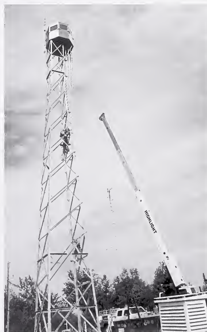
Flat Top Tower construction, raising 20 foot ladder section, Slave Lake Forest
